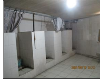
Photo of the sanitary facilities Toilet.JPG
