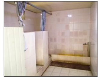
Photo of the sanitary facilities Toilet.JPG
